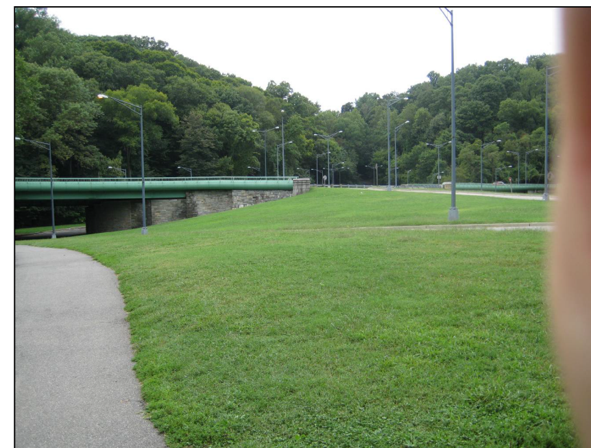
FIGURE 1 - LOOKING WEST TOWARD KLINGLE RD & PORTER ST NW INTERCHANGE
