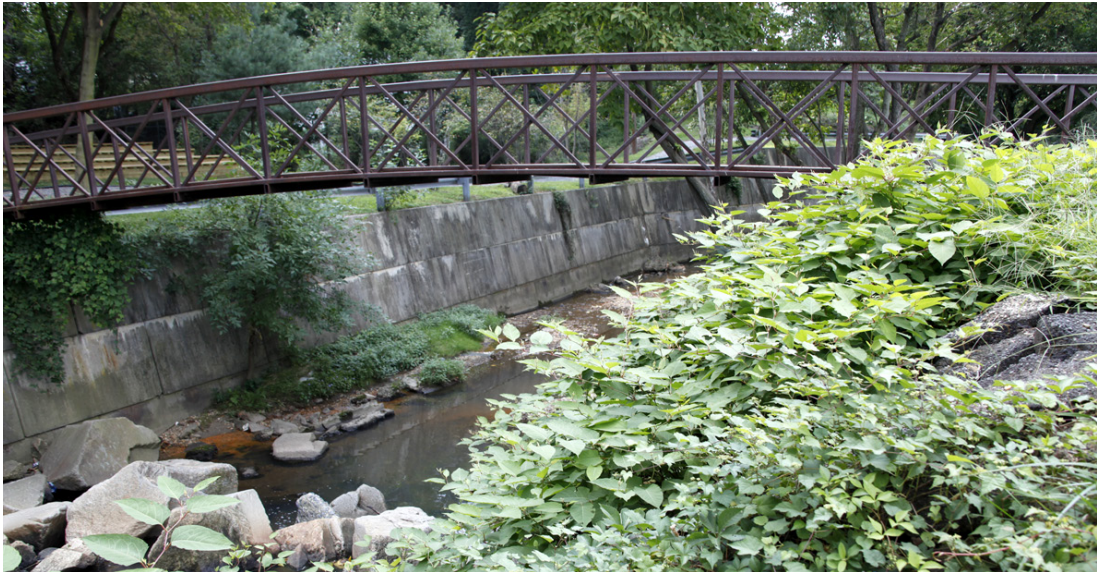
Pedestrian bridge at Marvin Gaye Park
