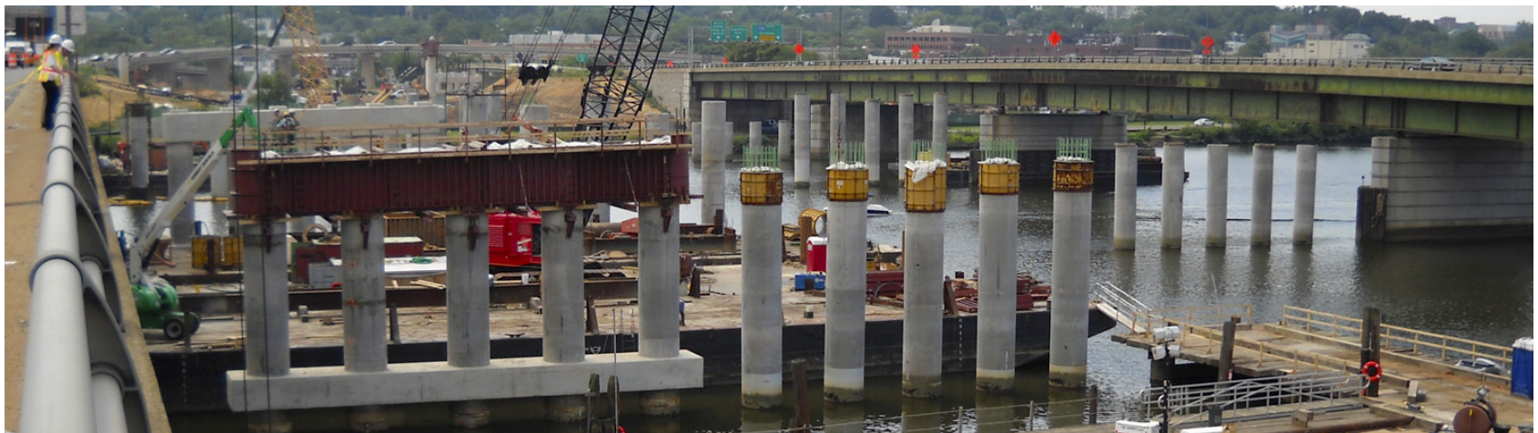
Construction on the 11 th Street Bridges
