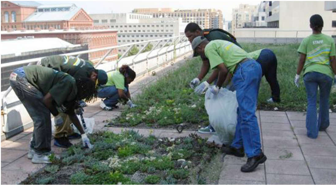
Volunteers planting a green roof
