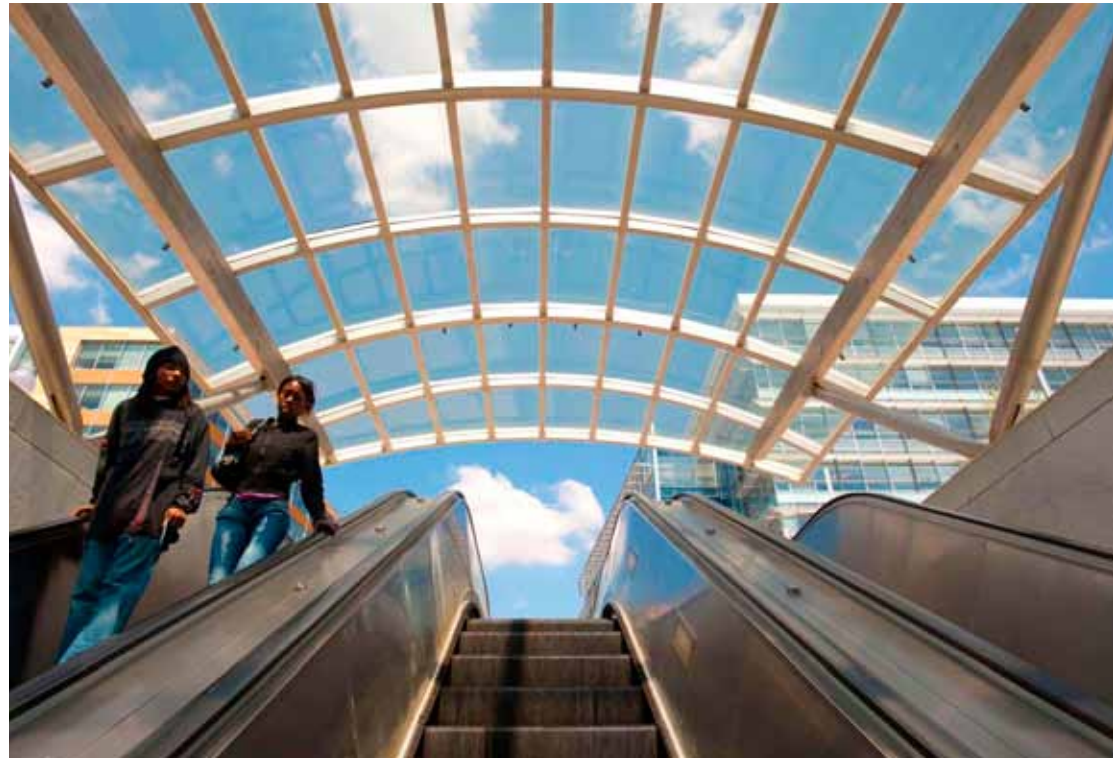
Waterfront metro station
