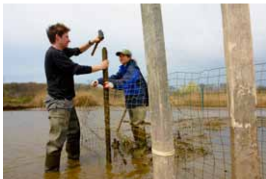
Constructing wetlands at Kingman Island
