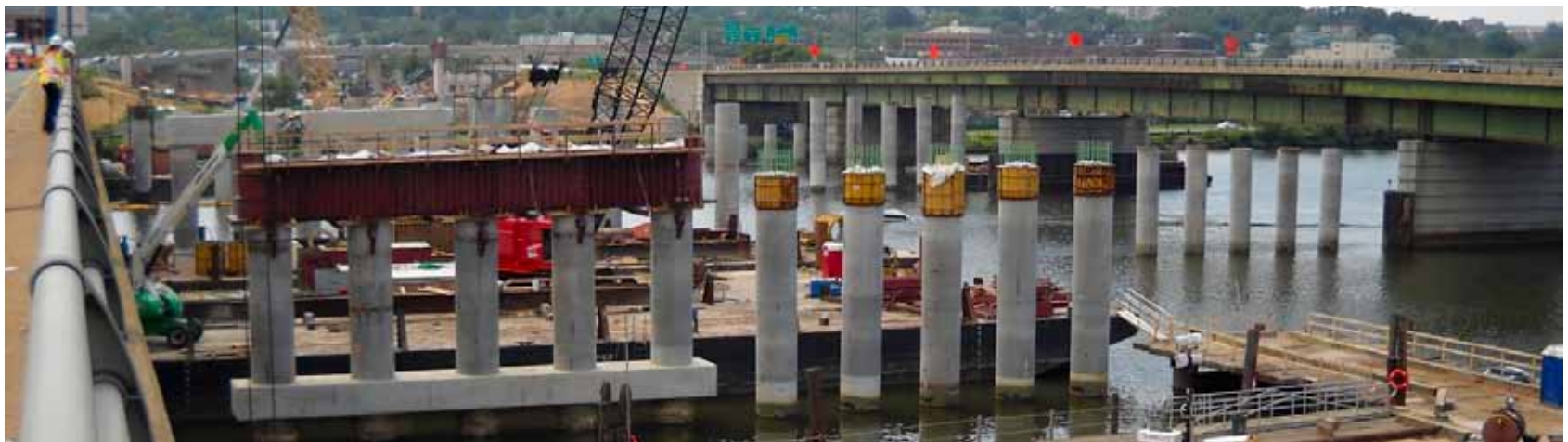
Construction on the 11 th Street Bridges
