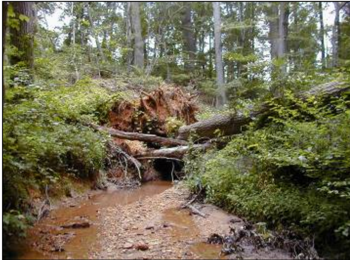
Severe Erosion, Ft. Dupont Tributary
