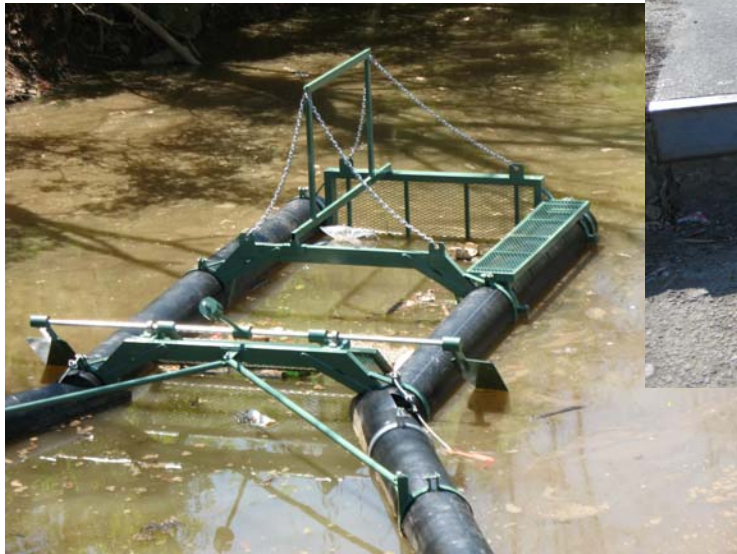
Bandalong trash trap in the Watts Branch watershed
