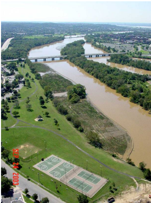
The River Fringe wetland adjacent to the River Terrace Community was created in 2003
