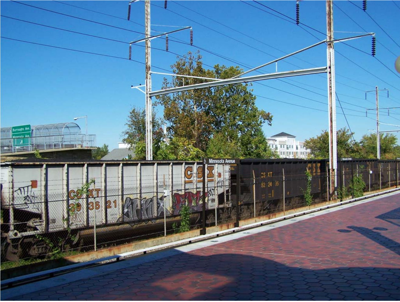
Utility Clearance at Minnesota Ave
