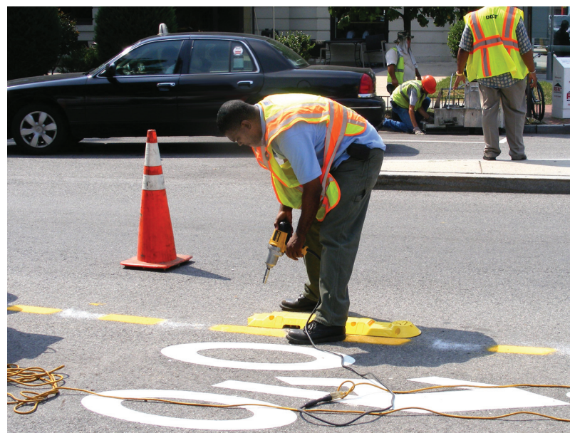
Top: Pedestrian rapid flash beacon; Bottom: DDOT worker installing bicycle pylon; Right: Pedestrians using raised crosswalk on E. Capitol St. NE (photo by Brandon Soublet)
