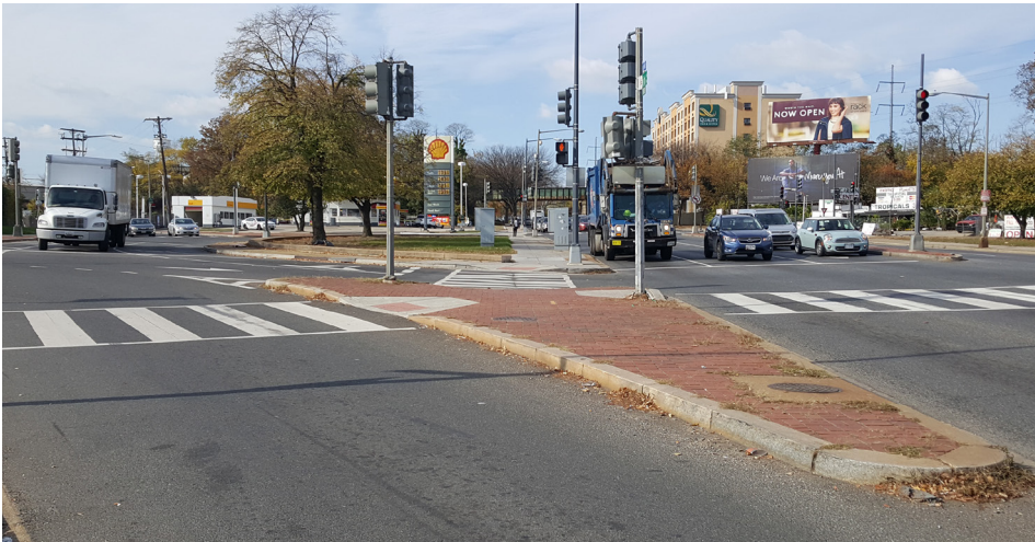
Photo 11: Existing crosswalk, curb ramps and refuge island at Montana Circle.
