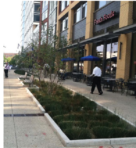
Photo 34: Example of bioretention planters along a Washington D.C. streetscape.
