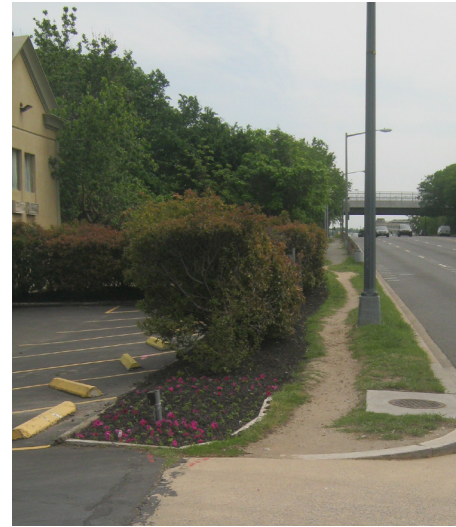
Photo 7: New York Avenue NE includes long stretches of areas with no sidewalk. Pedestrian worn, dirt paths have formed at these locations.
