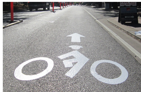
Photo 23: Shared Lane Markings
