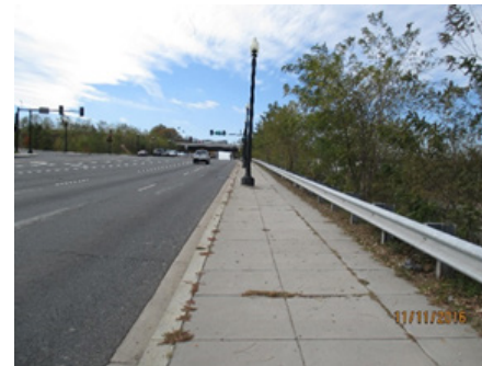
Photo 18: No tree pits exist at the 9th Street NE Bridge and New York Avenue NE Intersection.
